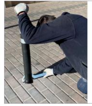
Screw the bollard with the help of the key (not included).
