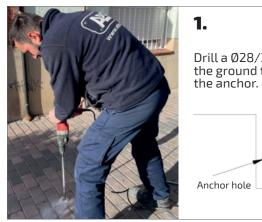
Drill a Ø28/30 hole in the ground to install
