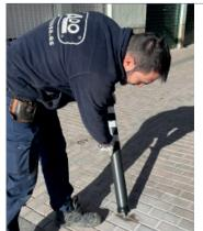
Let the resin dry (10 minutes) and then you can screw the bollard.
